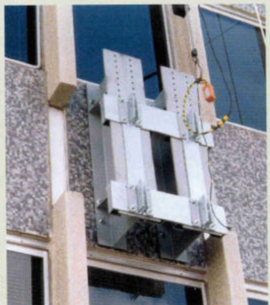
A specially designed mounting bracket placed the banner fabric about 0.91m (3 ft.) away from the vertical surface, creating a plenum air space.
