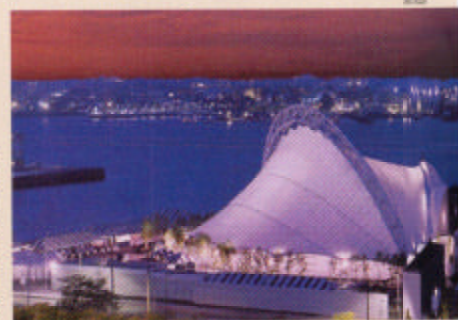
A finished pavilion glows in the night on South Boston's shores.
