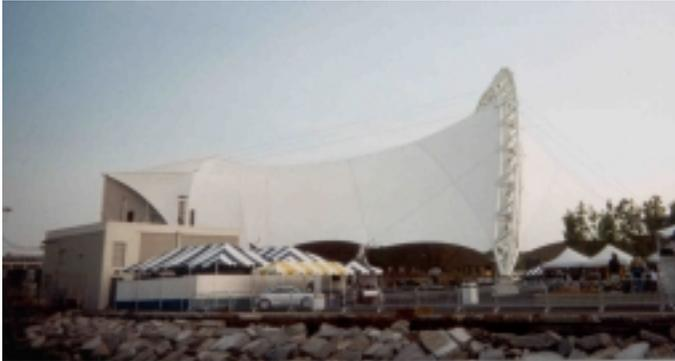
*Above:* The arch and tensile covering of the BankBoston Pavilion creates obstruction-free seating for all viewers. The stage house anchors the truss and roof.
