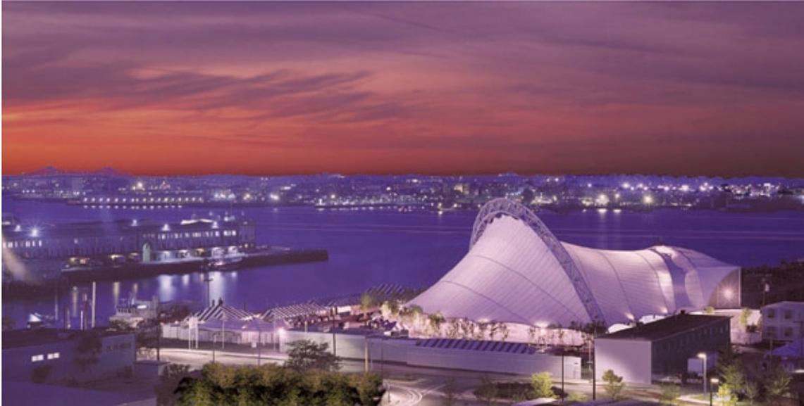
Designed by A.Form architecture pc, the BankBoston Pavilion is a 35,000 ft<sup>2</sup> tensile structure with seating for 5,200 persons. A mandate for, “obstruction free seating” lead to a single structural arch, 270 feet wide by 100 feet high. The arch scheme is most exceptional for interior views of the stage, and being the architectural identifying element of the facility’s exterior.
