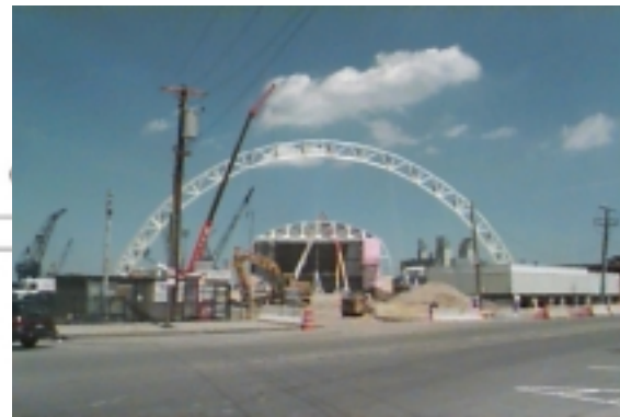
View of Stage House from Behind Main Arch
