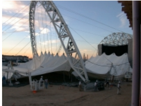
Arch and Stage House at Fabric Installation
