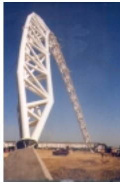
Arch and Foundation
