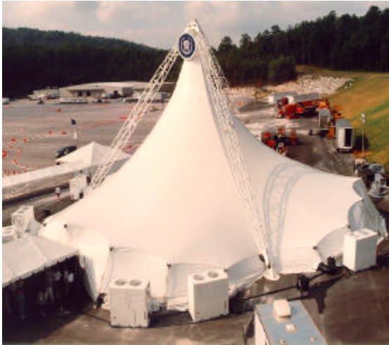
Top right: A plan view of the Pavilion illustrates the tripod structure which allows for an expedient assembly.
